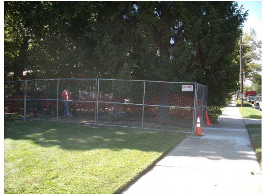
Chain link fence to secure the work zone
