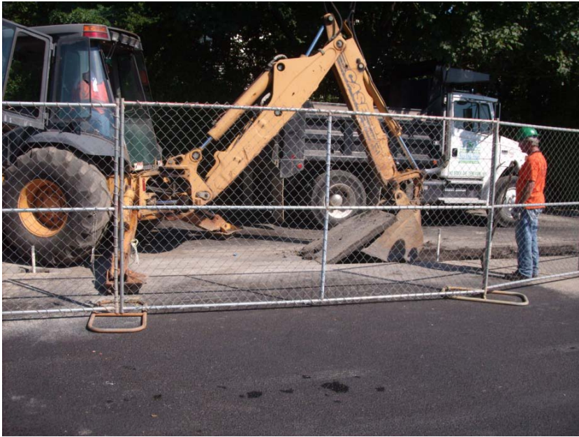
Trenching for HDPE injection lines
