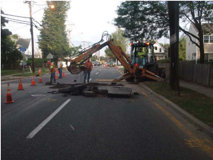
Trenching across left hand lane of N. Clinton Ave.
