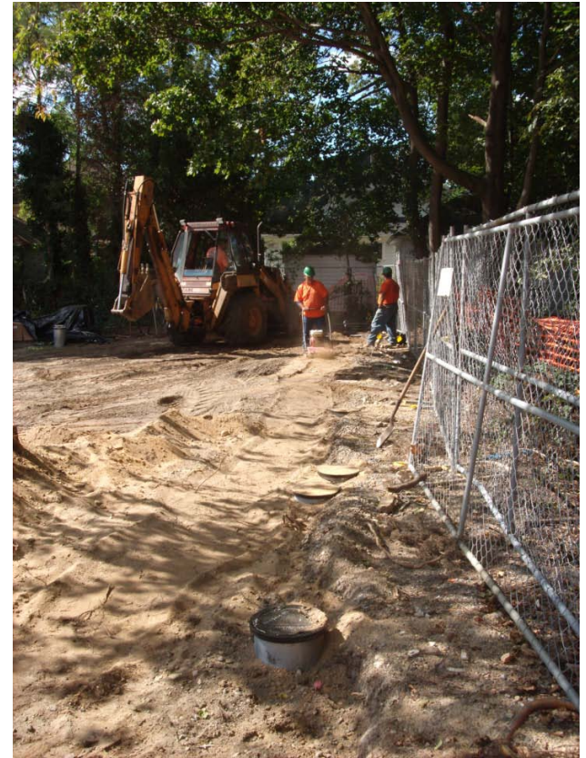
Trench backfilled to grade
