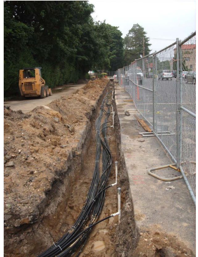
HDPE injection lines connected to injection point fittings
