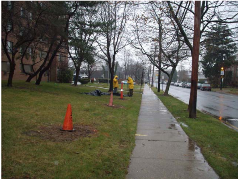
Hand clearing locations for injection points
