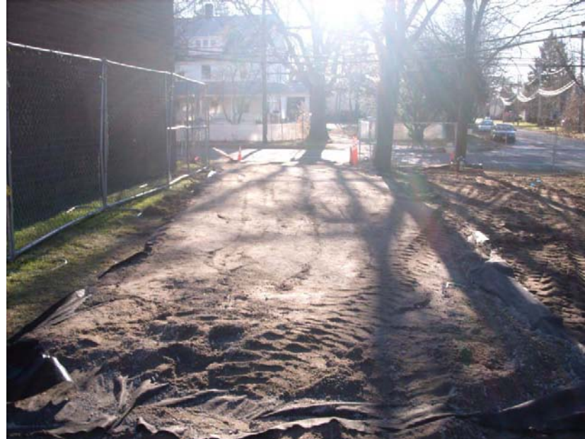
RCA Road for construction vehicles
