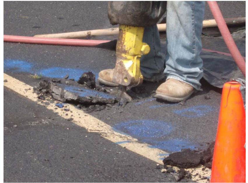
Breaking through asphalt to pre clear for injection point locations
