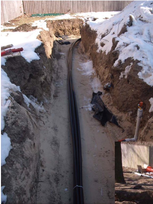
HDPE injection lines in NE portion of trench
