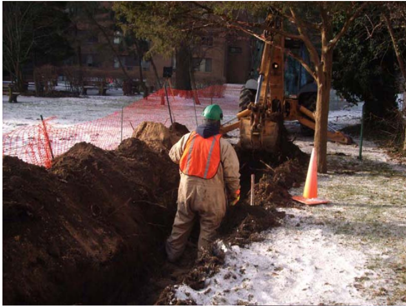
Trenching in NE corner of 33 N. Clinton Ave Property
