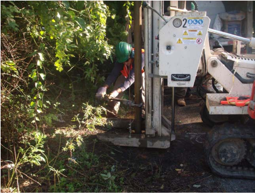
Installation of injection points
