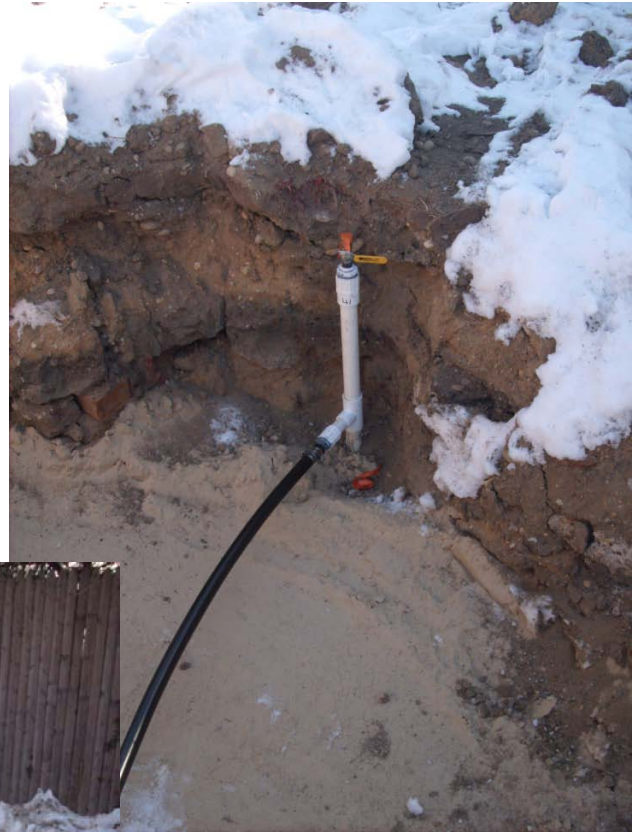
Injection point with fitting connected to HDPE line
