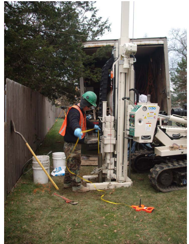
Installation of injection points
