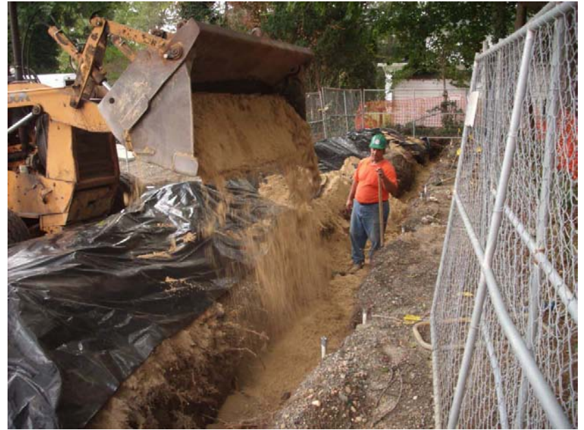
Backfilling the trench with clean material
