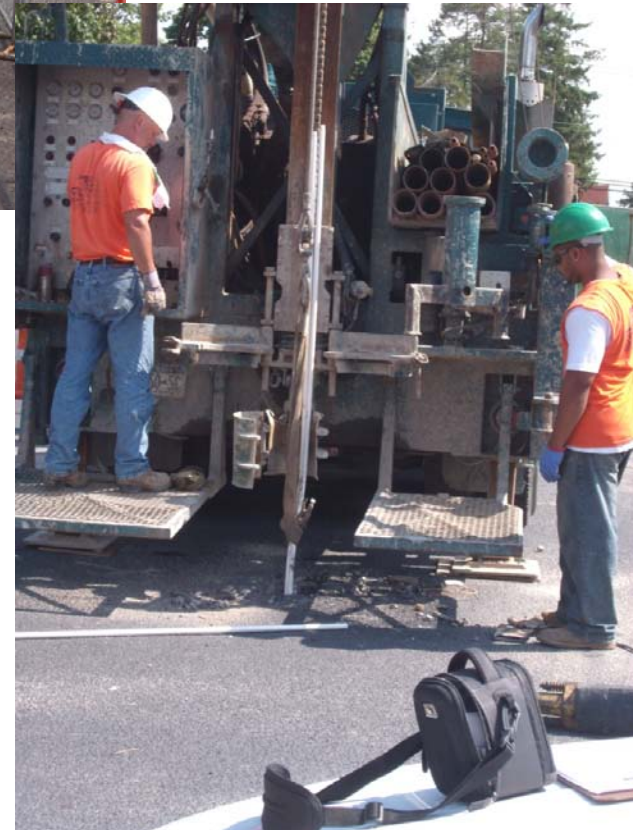
Abandoning county monitoring wells
