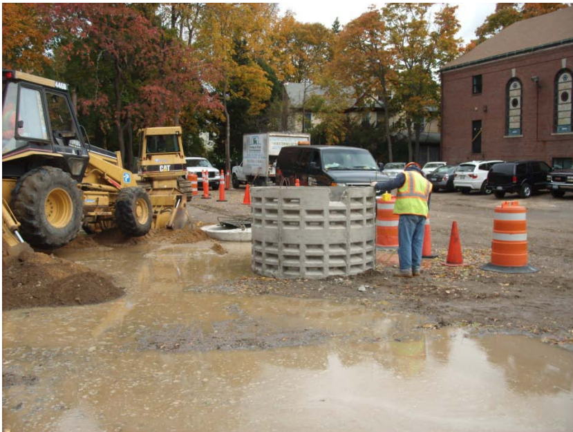
Installation of additional drainage in parking lot
