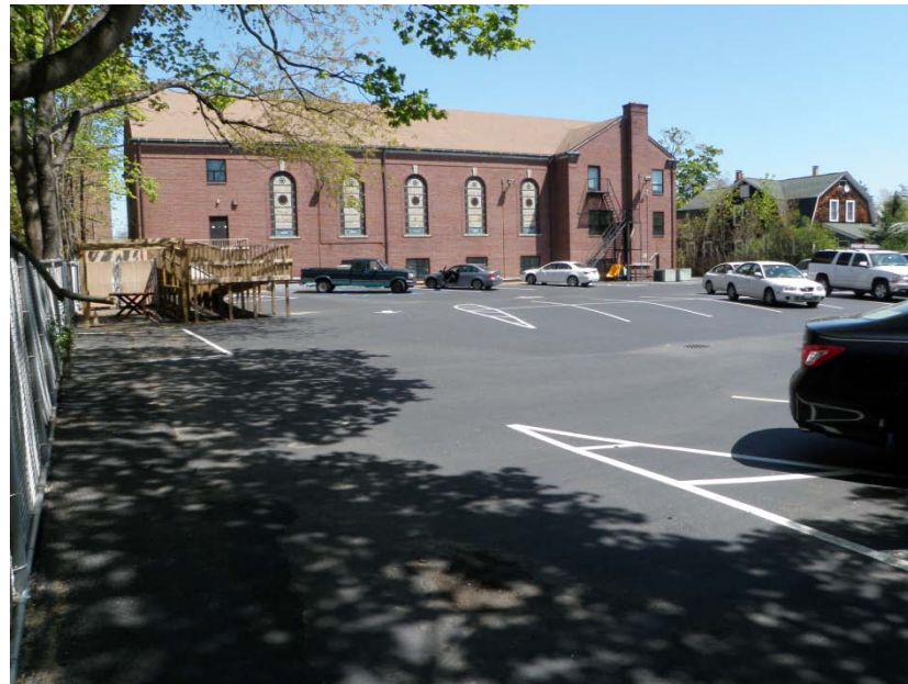
Restoration of parking lot
