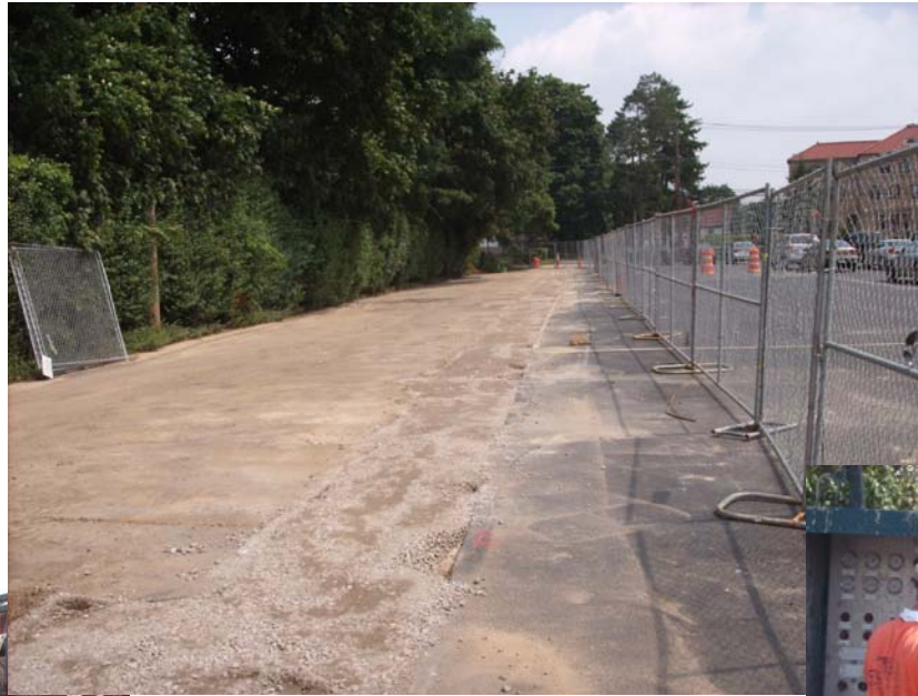
Trench backfilled to grade
