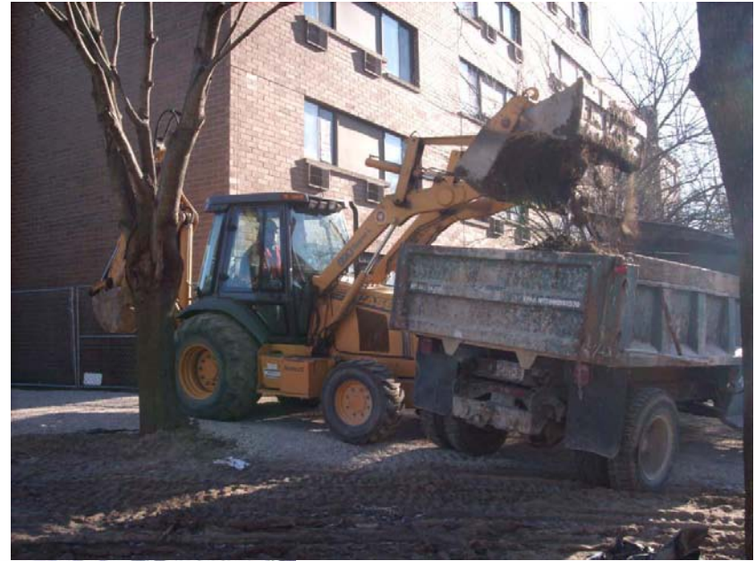
Trench soil debris removal
