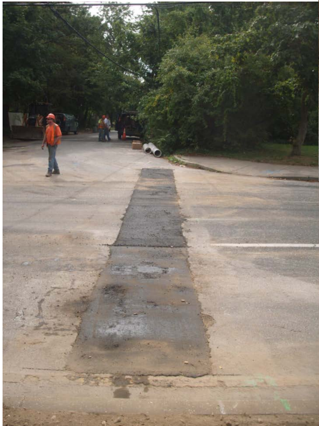
30 day temporary patching of N. Clinton Ave.
