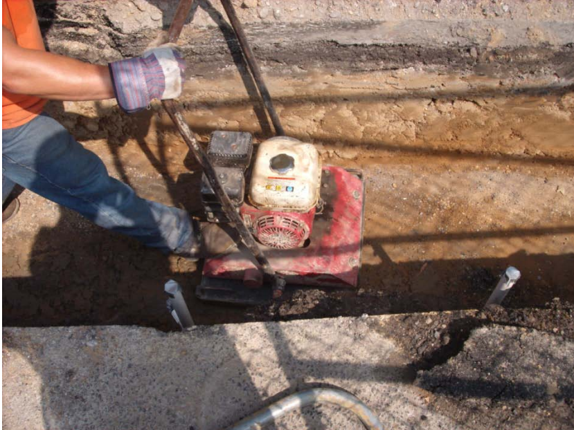
Compacting base of trench
