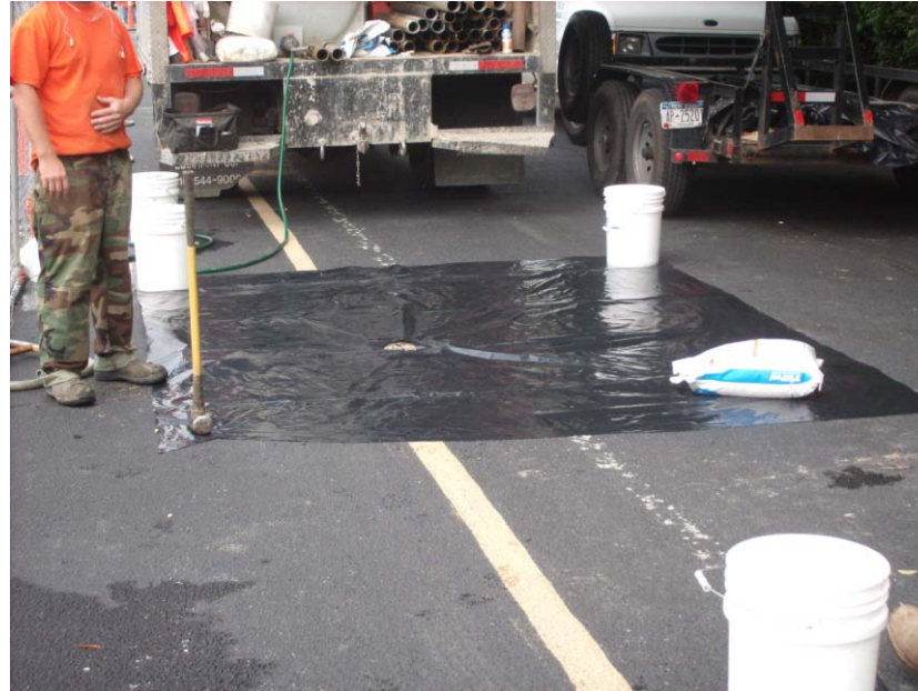
Preparing to install an injection point
