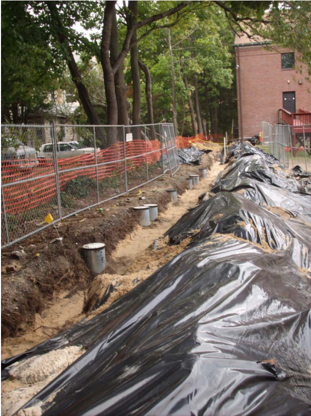
Erosion control of stock piled soil
