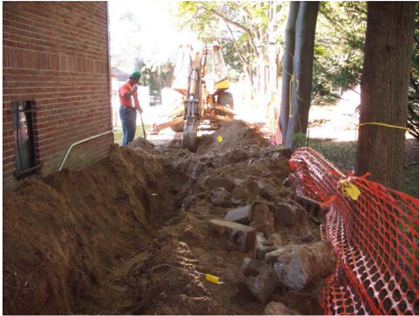
Trenching along northern property line
