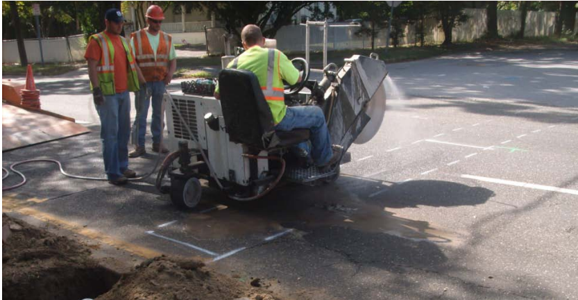
Saw cutting pavement of left hand lane of N. Clinton Ave.
