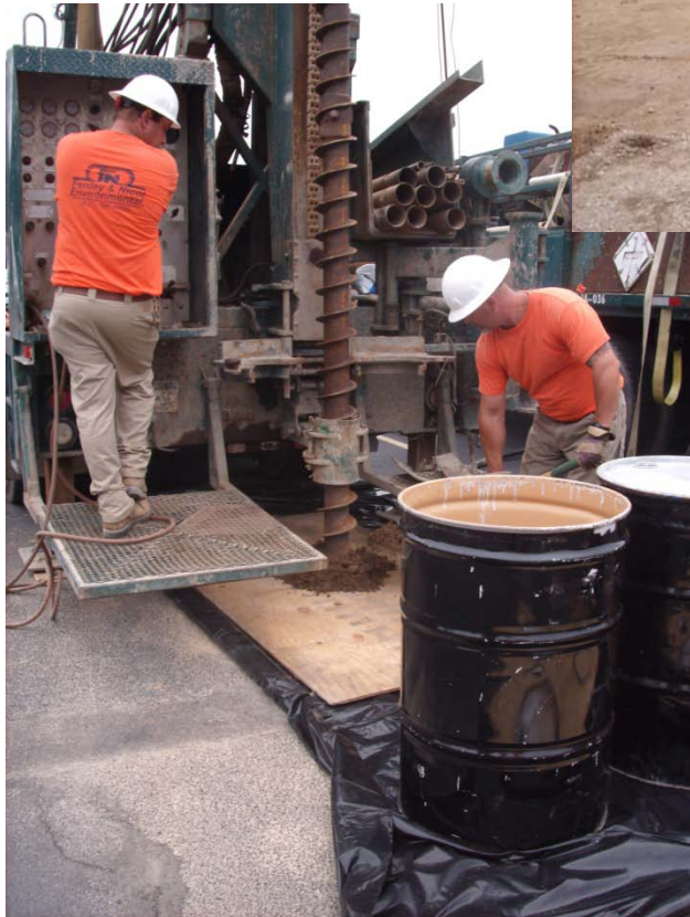
Installation of monitoring well cluster
