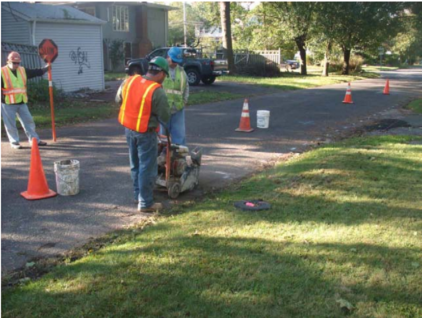
Saw cutting pavement for trench
