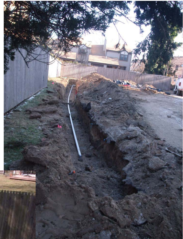
SVE line placed in trench in case needed in future
