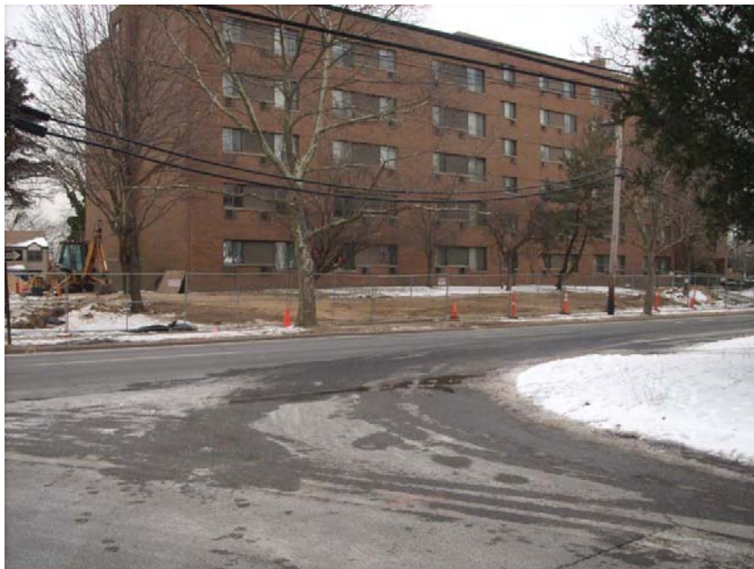
Chain link fencing to secure work zone
