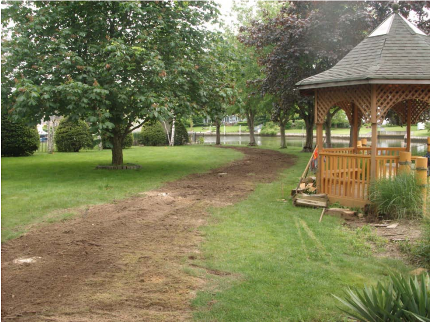
Trench backfilled to grade
