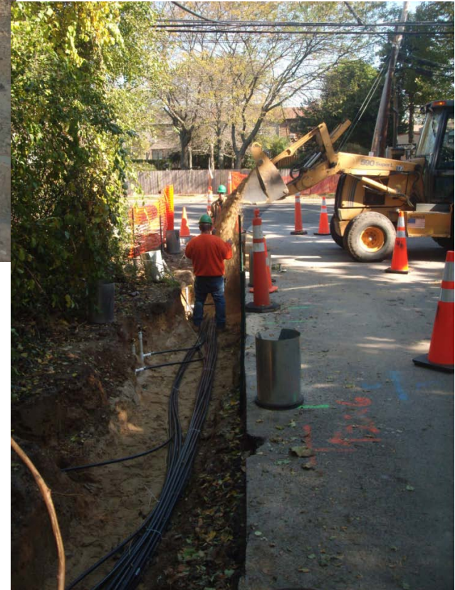
Backfilling trench with clean bedding sand
