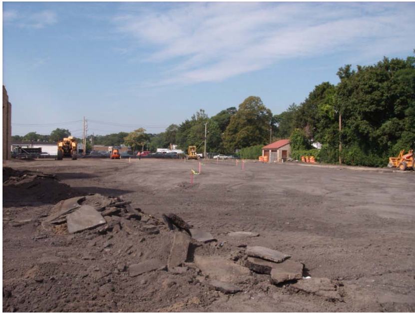
Pulverizing parking lot
