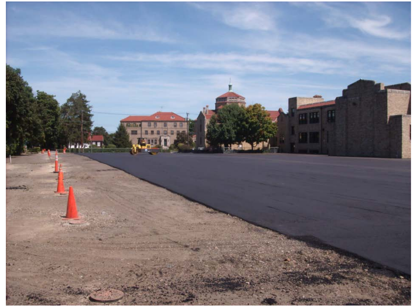
Paving parking lot
