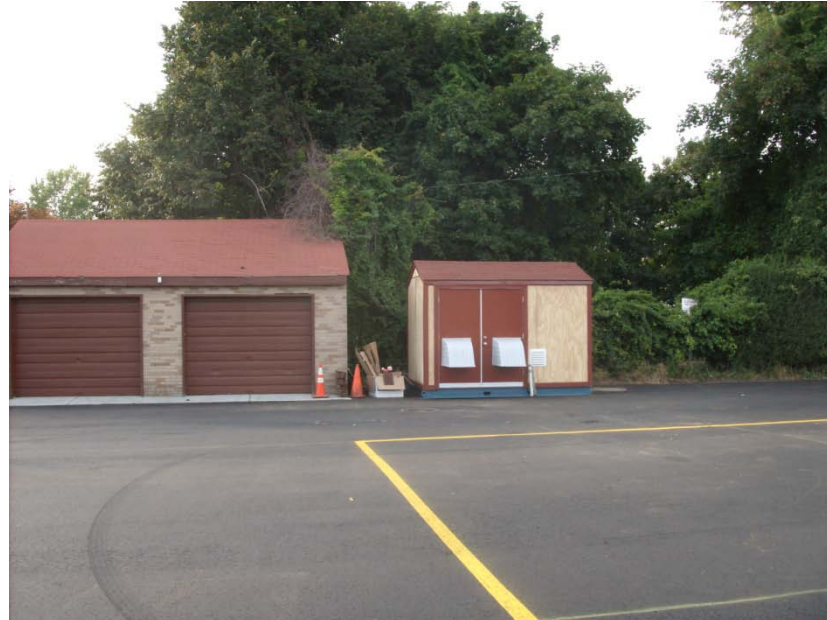
Oxygen Injection System Shed
