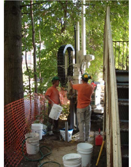
Injection point installation
