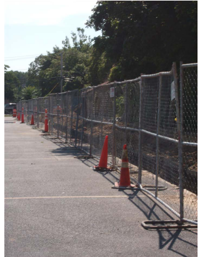
Chain link fence for containing the work zone
