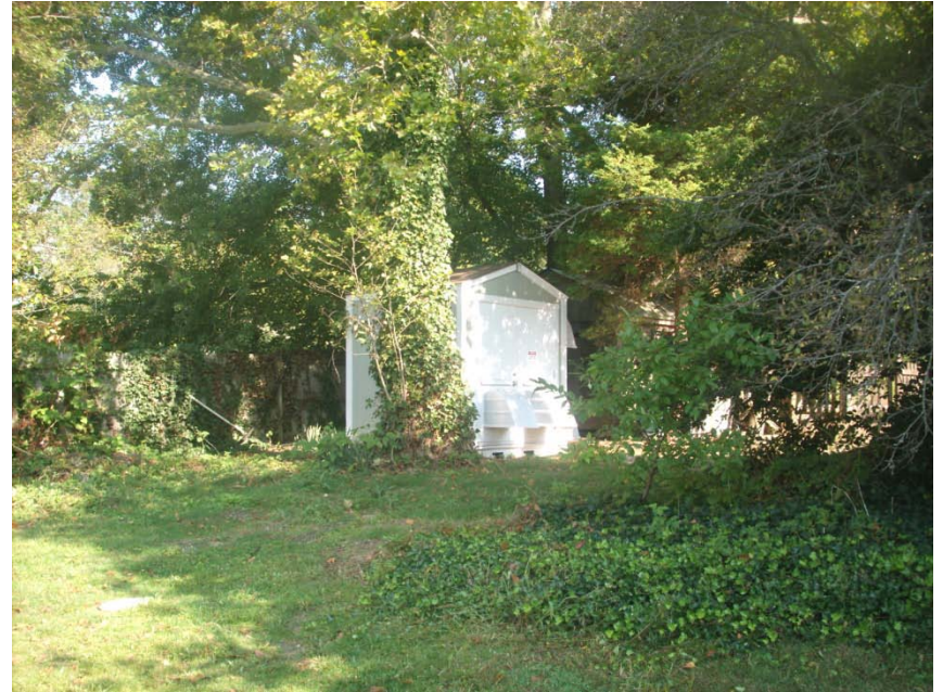
Oxygen injection system shed
