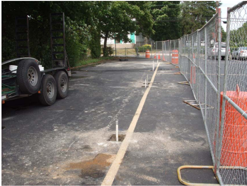
Installed injection points in NE corner of property
