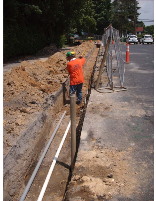
Backfilling above SVE lines
