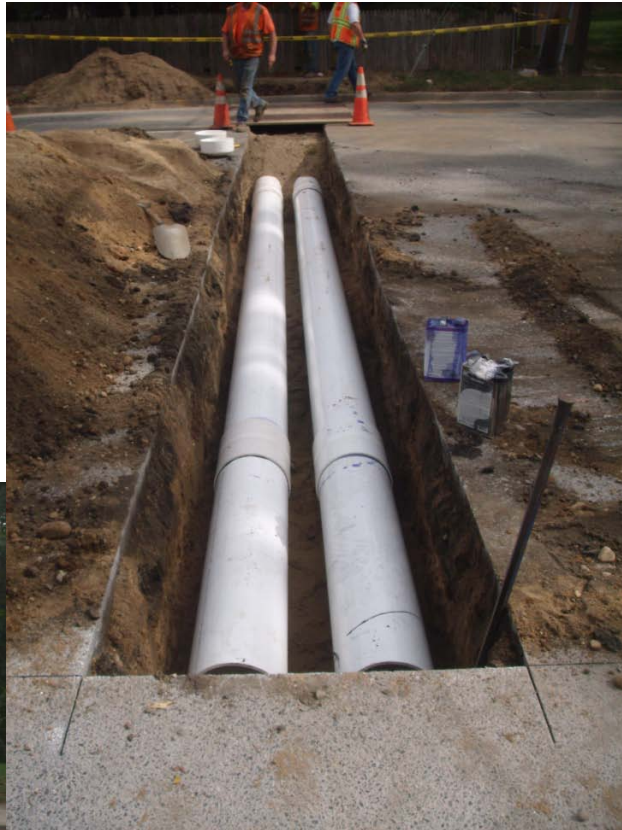
Placing conduit in trench of right lane of N. Clinton Ave.
