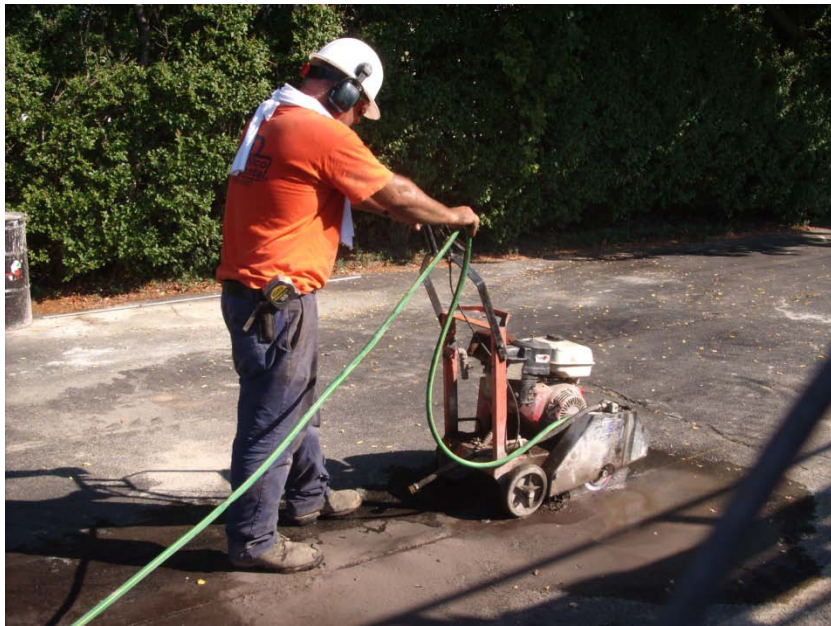
Saw cutting asphalt for trench location
